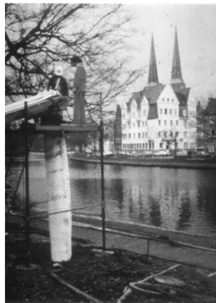
Damals: Inversion eines Liners DN 700 in Lübeck, Trave-Dükler
